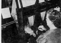
DRAWING IN—Operator pulls ends through needles.
